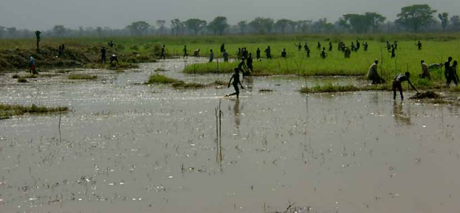
When the rainy season had come, dam workers and volunteers finished the last bits of work
