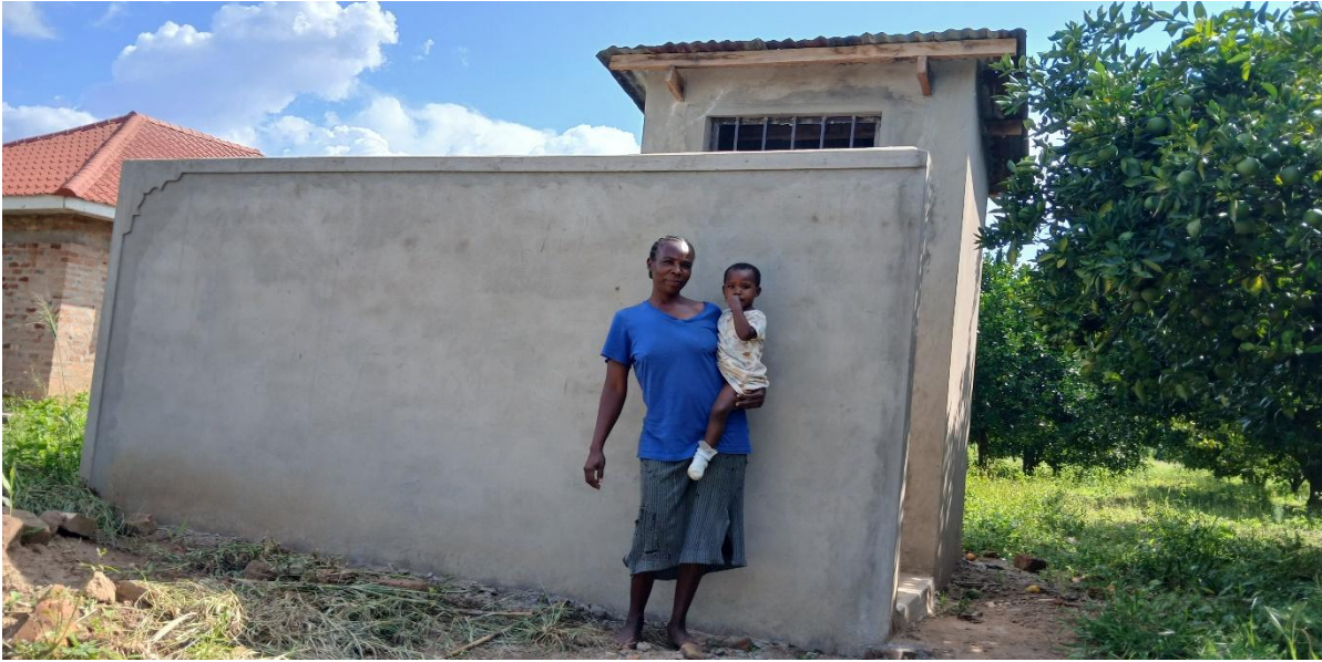
Adeke Dinah in front of her complete pit latrine
